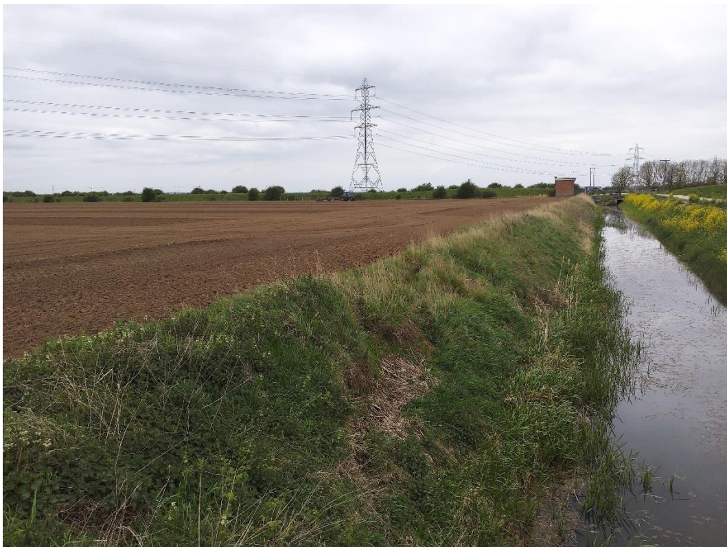
Bicker Drove looking towards pumping station and South Forty Foot Drain
